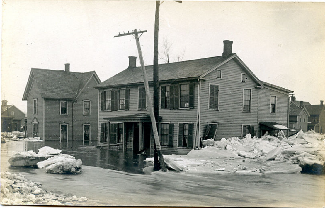
Flooded Residence, Ice Jam flooding, Herkimer, NY, undated
